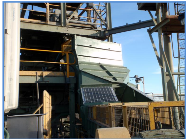
The new chute in position ready for commissioning
