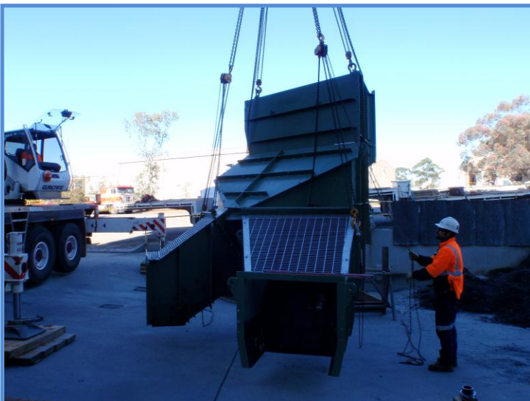
The chute arrival at Cobar CSA Mine ready for installation
